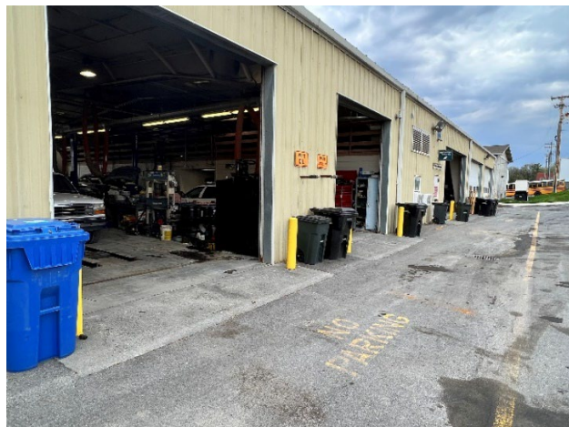
8 – Covered Trash Cans (Vehicle Maintenance Building)
