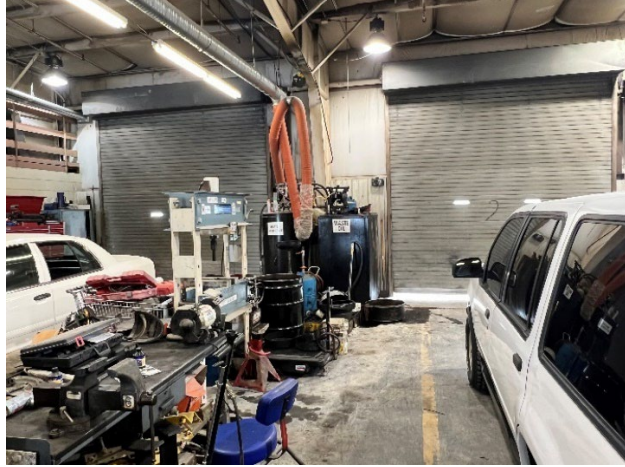
7 – Used Waste Oil and Antifreeze Storage (Vehicle Maintenance Building)
