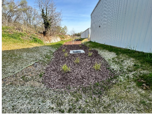
22 – Bioretention Outlet Structure
