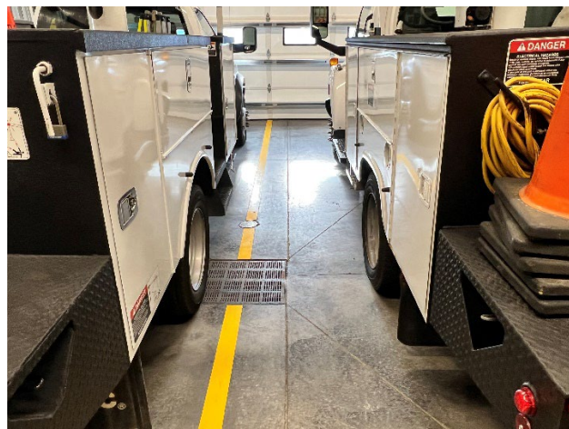
6 – Deck Drain (Building #4)
