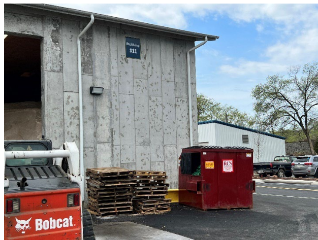
12 – Covered Dumpster (Building #11)
