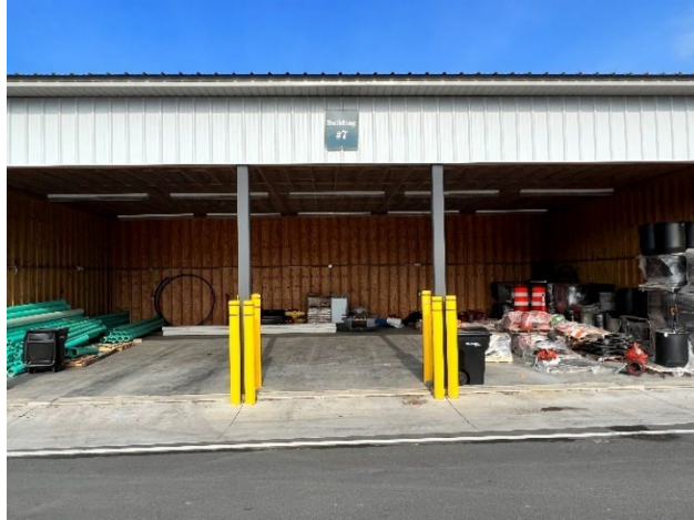
10 – Utility Maintenance Equipment (Building #7)
