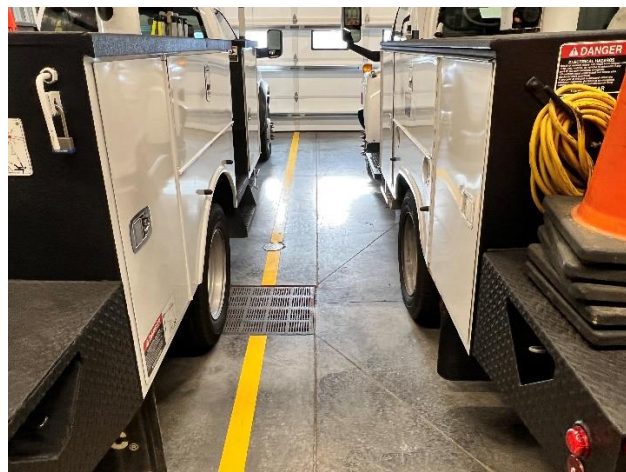
6 – Deck Drain (Building #4)
