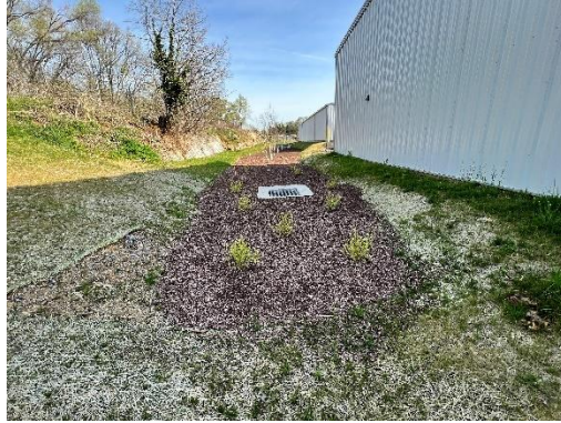
22 – Bioretention Outlet Structure
