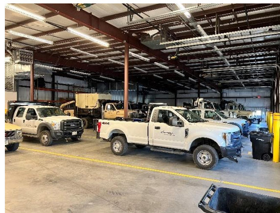
3 – Grounds Maintenance Equipment Storage (Building #2)
