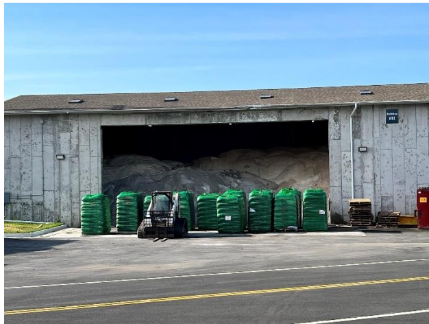
11 – Salt Storage Building (Building #11)
