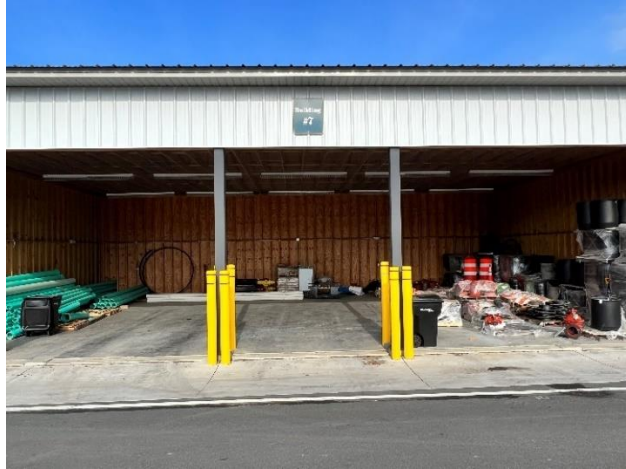
10 – Utility Maintenance Equipment (Building #7)
