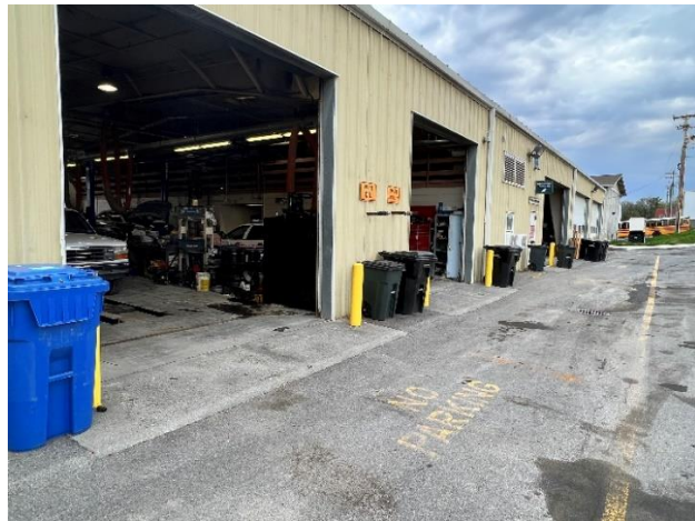
8 – Covered Trash Cans (Vehicle Maintenance Building)
